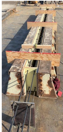
Figure 8: Formwork with stirrups and prestressing strands
