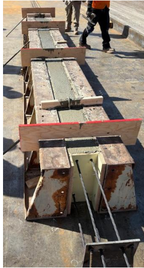
Figure 18: Beam after concrete poured
