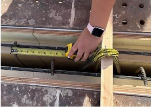
Figure 13 (left): Double lifting loop identifying side with 7 in. stirrup spacing
